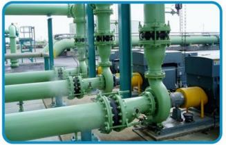
Elastomer expansion joints are characterized by gas tightness and drip tightness even if there is condensation.
